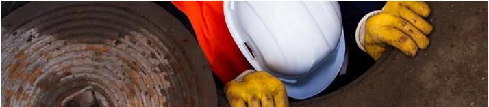
Confined Space" refers to a space which, by design, has limited openings for entry and exit, unfavorable natural ventilation which could contain or produce dangerous air contaminants, and which is not intended for continuous worker occupancy.
